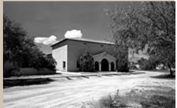
The Fulton-Hayden Art Gallery and Library, built in 1955, includes a 25,000 volume research library, meeting and classroom space. The Museum is to the left.
